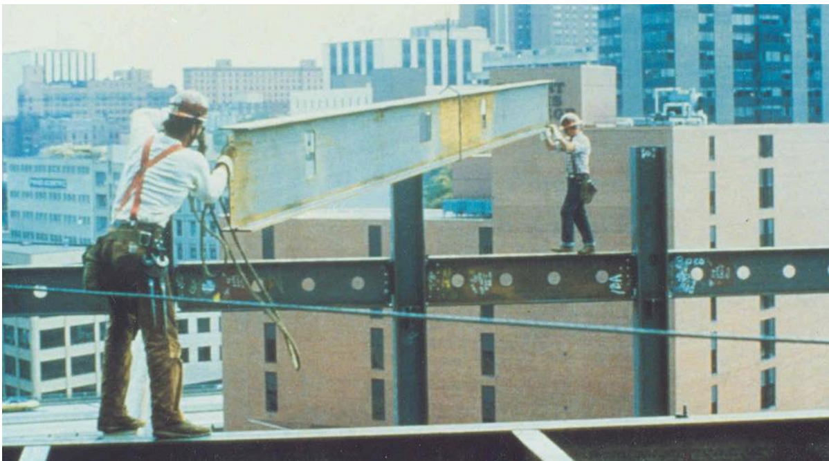
Fig. 7: Two iron workers wearing tool belts, while working at considerable height without fall protection equipment.
