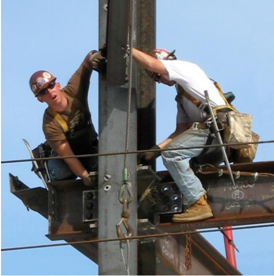
Fig. 5: Ironworkers erecting the steel frame of a new building, at the Massachusetts General Hospital, USA. Photo taken 2006
